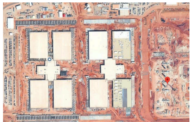
Satellite view (Google Maps) of two data centers at OpenAI’s Stargate I site in Abilene, Texas. The red marker indicates the gas-fired generators.
