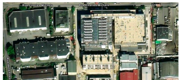
Satellite view (ESRI) of the Equinix PA12 expansion site in Argenteuil
